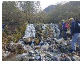
Ken-ei Sabo, Stone-pile check dam (Built 1906- 1926)
