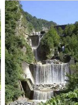
②Shiraiwa Sabo dam (Built 1929 - 1939)
