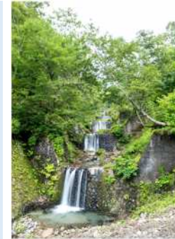
①Dorodani Sabo dams (Built 1930 - 1938)
