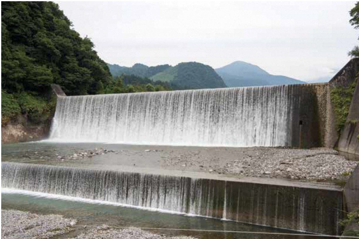
Hongu Sabo Dam
