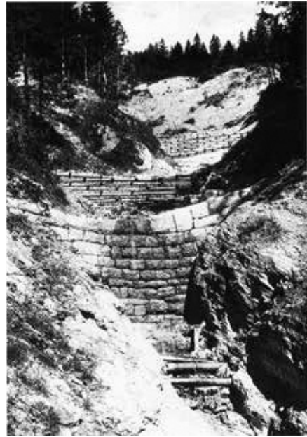
Check dams in Emsbach, Hohenems, Austria (1902)
