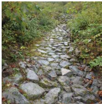
Stone-pile spillway in Nishinotani
