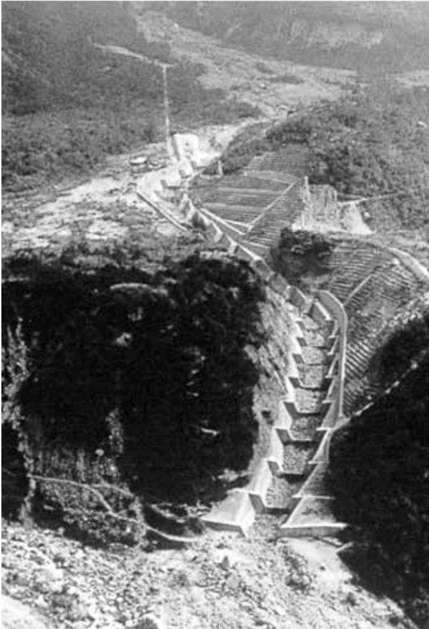
Immediately after the completion of the Dorodani Sabo Dams by Ministry of Home Affairs (1933)
