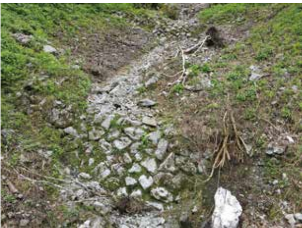
Stone-pile check dam in Nishinotani
