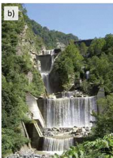
b) Shiraiwa Sabo Dam (Tallest Sabo dam in Japan : 108m) Built from 1929 until 1939 Function: - Fixing unstable sediment
