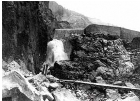
Yukawa No.1 Sabo Dam
