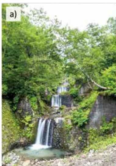
a) Dorodani Sabo Dams (22 dams) Built from 1930 until 1938 Function: - Spillway on unstable sediment - Erosion prevention - Reforestation
