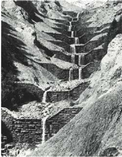
Check dams in Bretter Wantbach, Matrei, Osttirol, Austria
