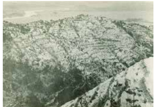
Hillside works at Tanakami area (Photo taken in 1908)
