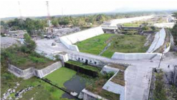
Indonesia : Sabo dam in Mt.Merapi (Courtesy of Yachiyo Engineering Co., Ltd.)
