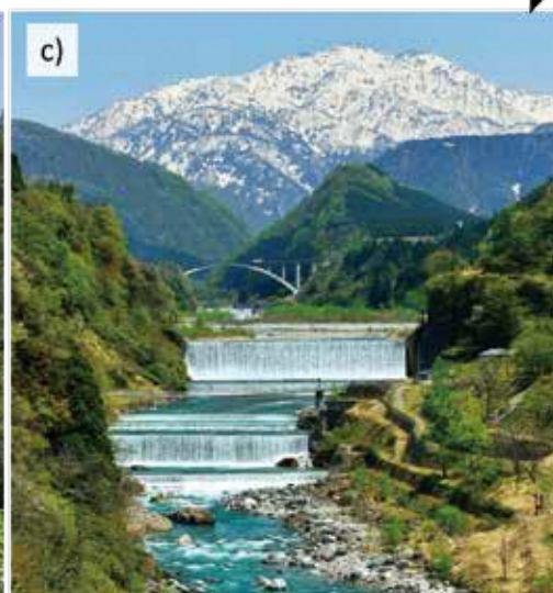
c) Hongu Sabo Dam (Largest storage volume : 5 million m 3 ) Built from 1935 until 1936 Function: - Temporal storage of sediment
