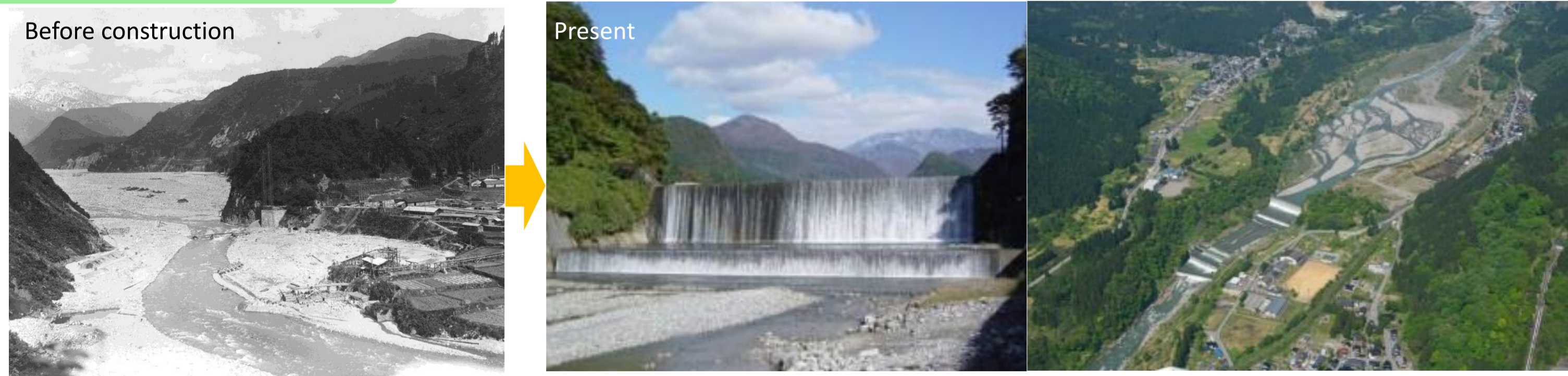
Fig.6 Changes of The Hongu Sabo Dam
